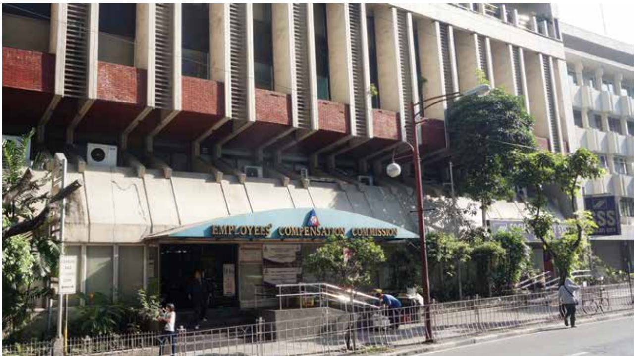
Employees' Compensation Commission (ECC) Building, 355 Sen. Gil Puyat Avenue, Makati City
